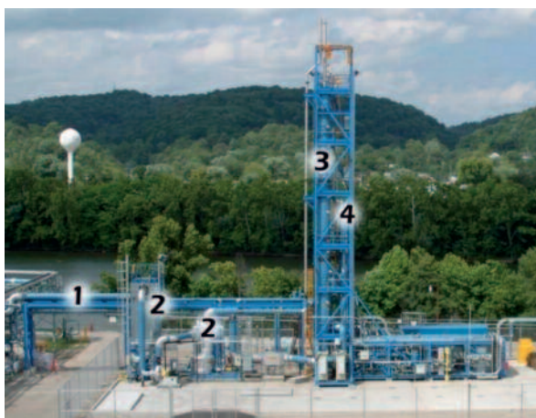
Figure 9. — The Charleston DOW – ALSTOM pilot CO 2 capture plant in West-Virginia, USA (post-combustion capture, http://dow-alstom.charlesryan.com )
