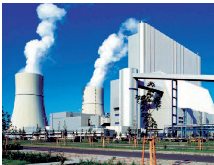
Figure 10. — Schwarze Pumpe in Germany. This power plant by Vattenfall has a 30MW th pilot oxyfuel capture plant ( www.vattenfall.com/www/co2_en/co2_en/index.jsp ).
